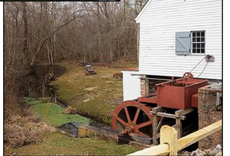
The water wheel, pictured above, turns because of the water flowing underneath of it. The wheel is connected to gears and conveyor belts, or elevators, inside which take grain up to the grinding wheels.
